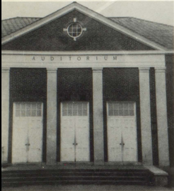
Entrance to the Auditorium.
