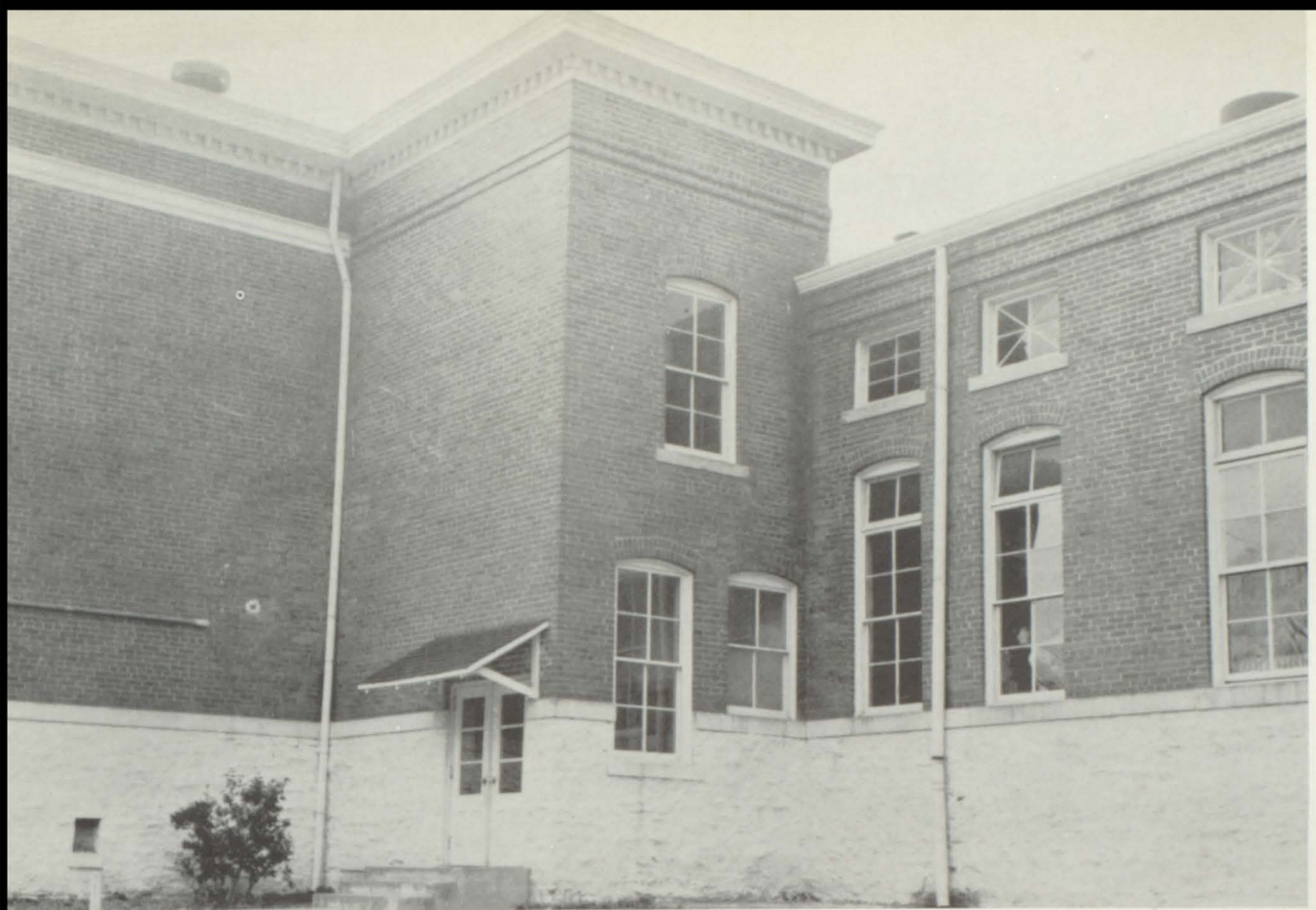
Pictured above is a side view of Old Main at CHS. Below is a view of the Agriculture and Home Economics Building.
